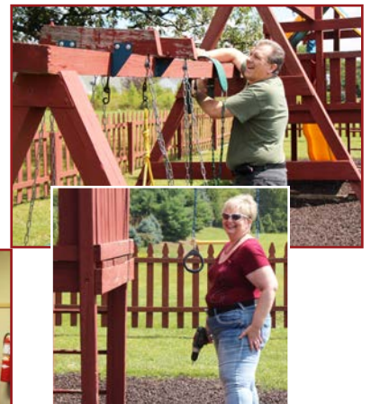
At left, Dan Brill, Larry Cooper and Carlo Cherubini repair the Sacristy cabinet after it was moved to make way for new carpet. Above, Chris and Cherie Bryant shore up the playground.
